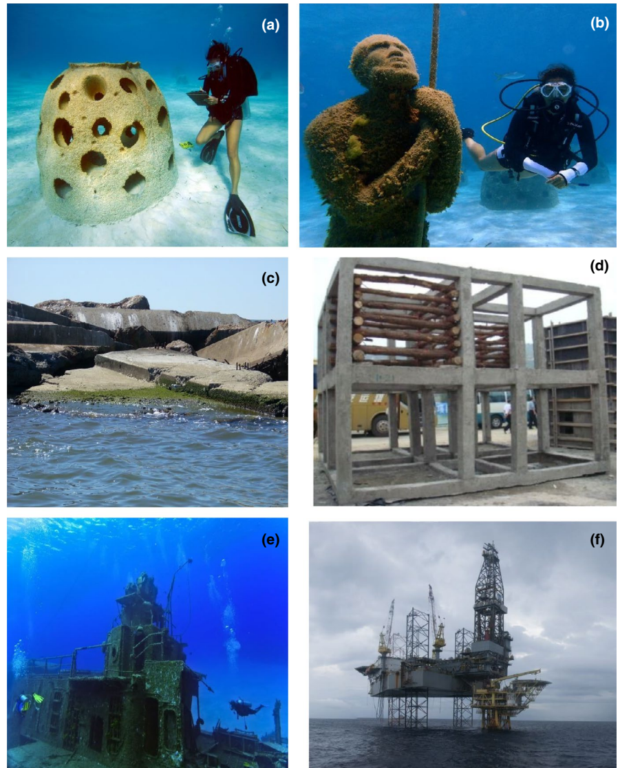
FIGURE 1 Structures that fall within a broad classification of artificial reefs: (a) a reef ball immediately after deployment on New Providence Island, The Bahamas; (b) one of the pieces in the Sir Nicholas Nuttall Coral Reef Sculpture Garden, New Providence Island, The Bahamas; (c) Katrina Reef off the coast of Mississippi, made of limestone and crushed concrete—see Mazzei and Biber (2015); (d) one component of an artificial reef complex deployed in Daya Bay, China—see Yu et al. (2015); (e) the Tibbetts, a Russian frigate that was sunk in the waters of Cayman Brac, Cayman Islands and (f) oil and gas platform in the South China Sea. Photograph credits are listed in Acknowledgements
